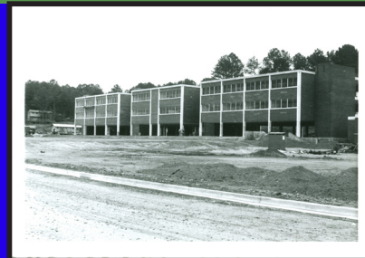
Photograph showing final stages of the construction of the Ashford-Dunwoody campus of Marist School in July 1962.
